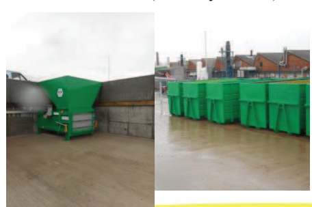
Household Waste (service yard side)
